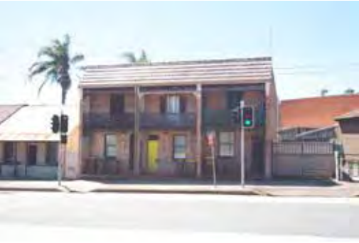
6 Residential Properties on Victoria Road
